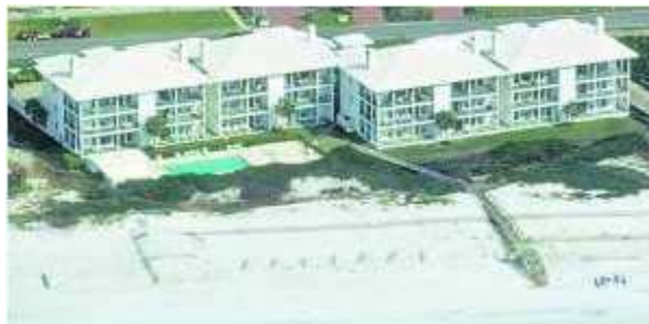
Picture of building at issue in file # FR-878 AR ATF
